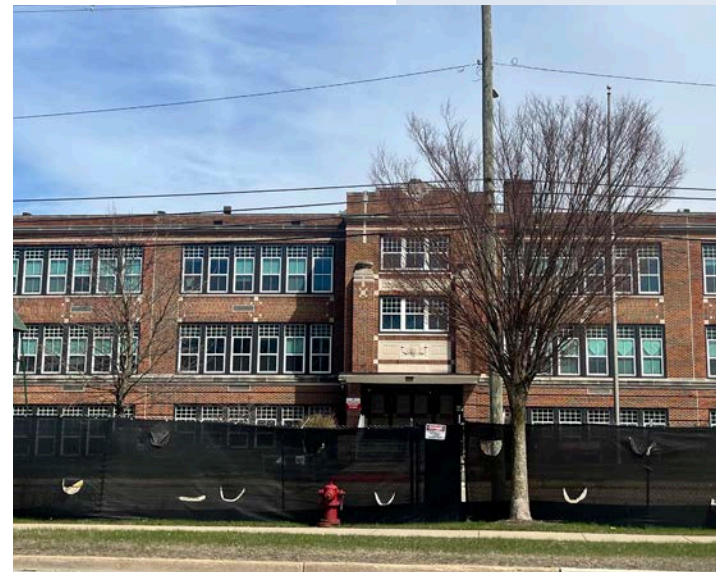
Figure 5.4 Roosevelt Elementary School as pictured in April 2025.
